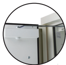
Self-closing door(s) with thermo-fuse
