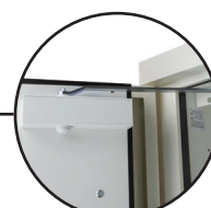
Self-closing door(s) with thermo-fuse
